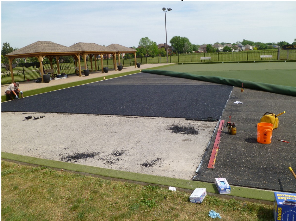
Photo taken on May 29, 2016 during repairs to base
